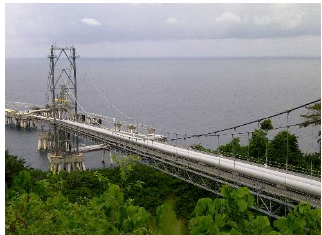
Natural gas pipe rack suspension bridge in Punta Europa, Equatorial Guinea (Source: Reuters)
